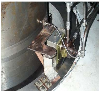
Eddy Current Probe for Shaft Position
