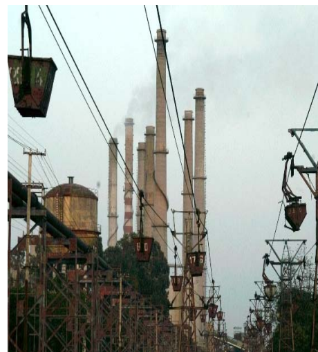
Figure 4 Taking Coal to the Power Plant
