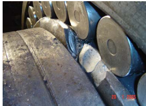
Figure 10: Converter Bearing – Detected at 1.5 rpm
